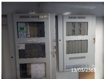
Fire Alarm Control Panel
